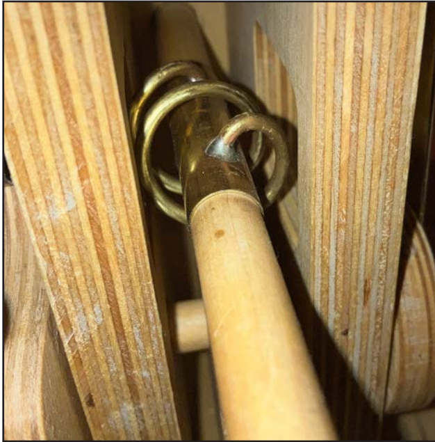
5. A brass worm is soldered to a brass sleeve over the wooden shaft for greater security.
